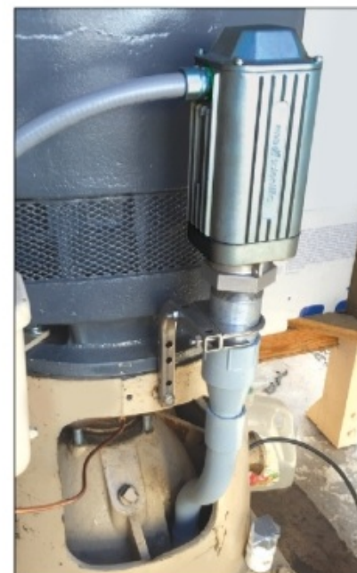
Smart Probe installs at the well cap with 2" NPT(F) threads.
