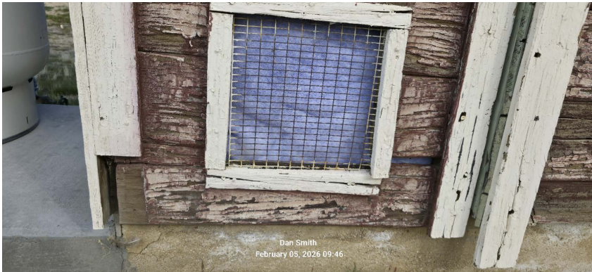
Air vents/windows are now covered with a mesh filter to prolong the VDF electrical panel components
