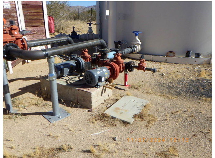
Figure 17: Booster pumps
