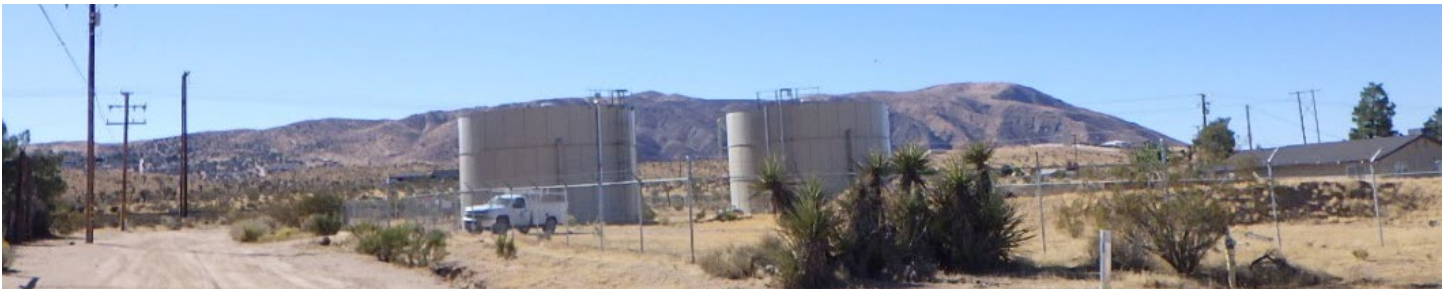
Figure 11: Thompson Family East & West Tanks
